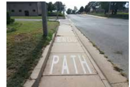
Discontinuous Path along Academy
