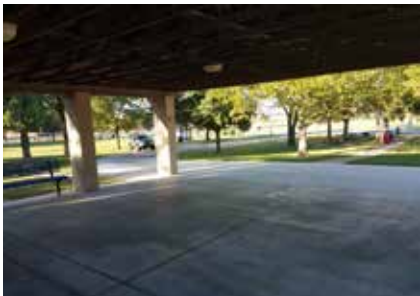
West Side of Community Building
